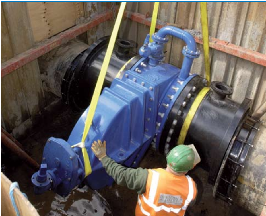
Upgrading mains serving Newcastle upon Tyne.
