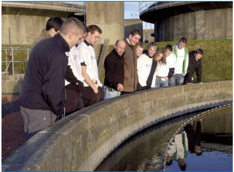
NWL's apprentices visiting Birtley sewage treatment works near Gateshead.
