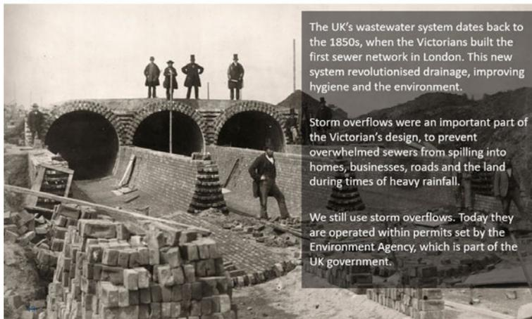
The UK's wastewater system dates back to the 1850s, when the Victorians built the first sewer network in London. This new system revolutionised drainage, improving hygiene and the environment.
